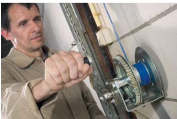
Raising the water lines
